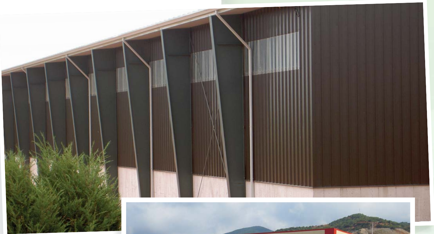
Above: The exterior columns provide a natural overhang on the building as well as a unique look.
