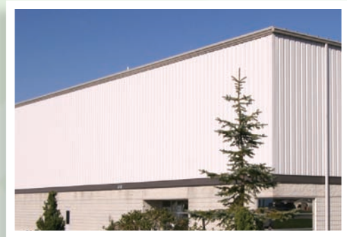
A custom accent band is used in the transition from masonry to steel cladding.
